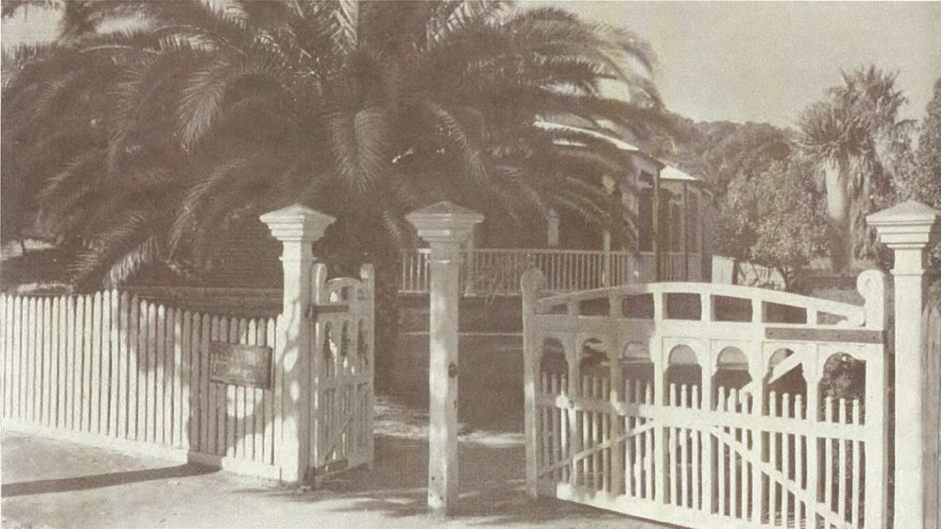
1940, from View Street gates:
