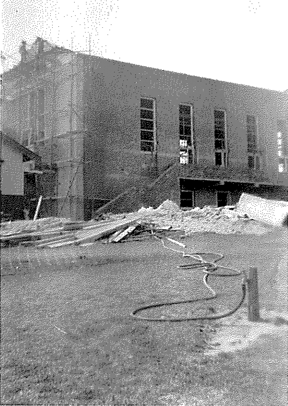
Construction of Carmichael Hall, 1954-1955:
