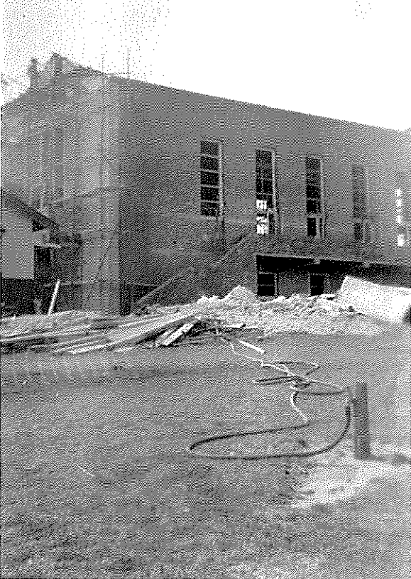
Construction of Carmichael Hall, 1954-1955:
