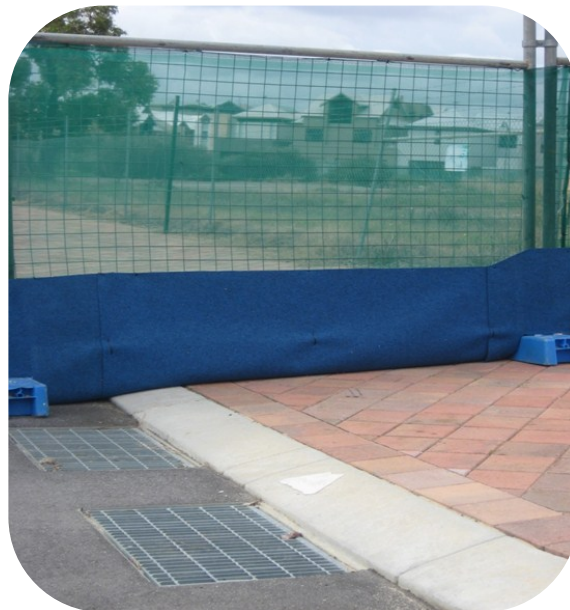
Figure 2: Front view showing sediment control fence protecting stormwater drains
