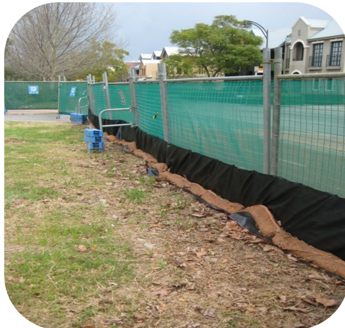
Figure 3: Side view showing fence with geotextile fabric secured to the ground
