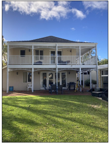
PHOTO 02 AND PHOTO 03 EXISTING TIMBER ENTRY PERGOLA TO BE DEMOLISHED
