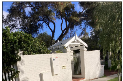
PHOTO 01 EXISTING TIMBER ENTRY PERGOLA TO BE DEMOLISHED
