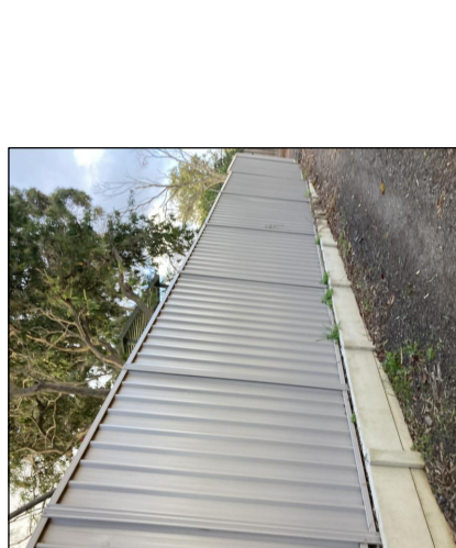
PHOTO 08 AND 09 GARAGE AND SURROUND LANDSCAPING TO BE DEMOLISHED AND REMOVED
