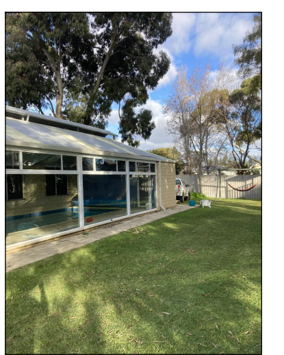
PHOTO 05 EXAMPLE OF EXISTING TIMBER GLAZING PROPOSED TO BE REPLACED WITH STEEL FRAMED GLAZING
