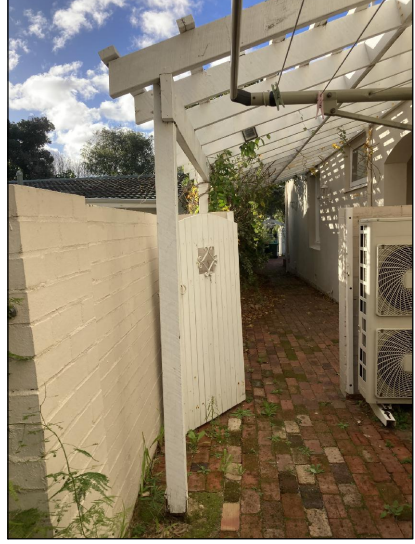
PHOTO 04 TIMBER PERGOLA TO SIDE OF ORIGINAL COTTAGE TO BE REMOVED
