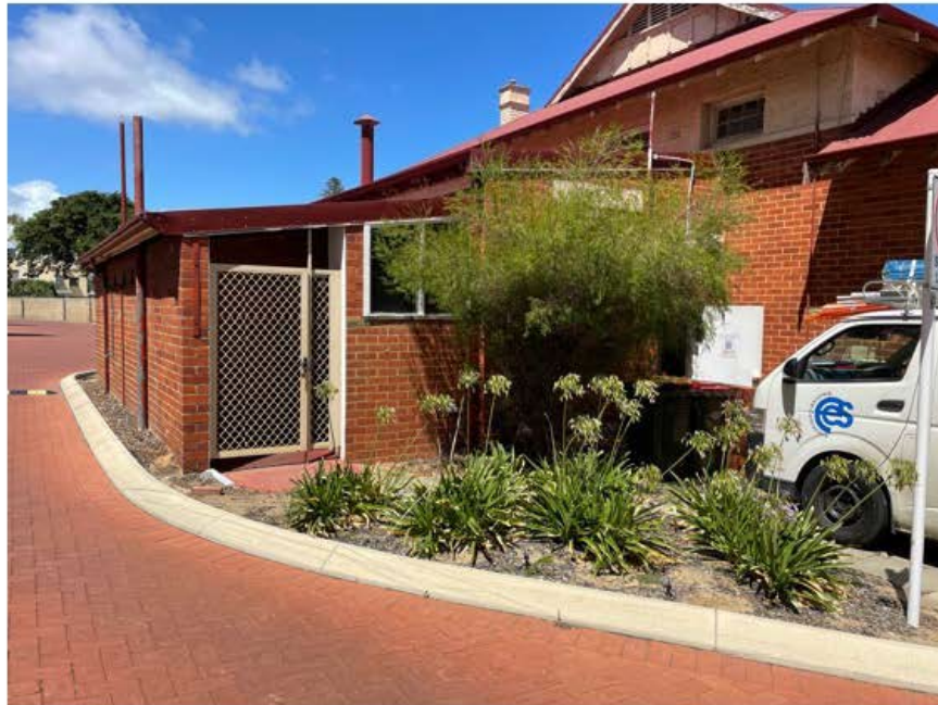
Photograph D4: The toilets at the rear which are intrusive. They have been modified, added to and no longer meet NCC requirements. Griffiths Architects February 2022
