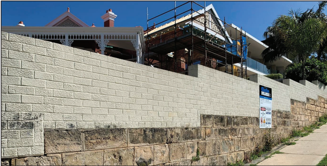
Photograph 7: The existing boundary wall of the subject site, as viewed from The Esplanade verge.
