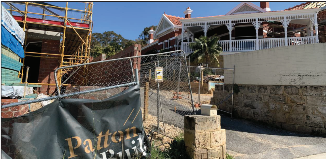
Photograph 8: The existing boundary wall of the subject site, as viewed from The Esplanade verge.
