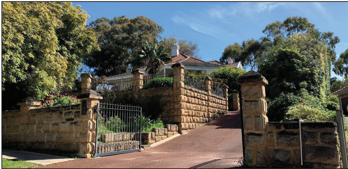
Photograph 1: Solid 'Pillow Face' limestone front walls at No.150 Forrest Street, with terraced landscaping and open fencing above.
