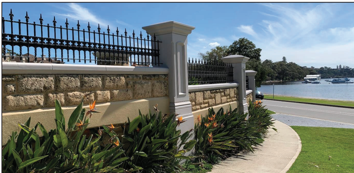
Photograph 6: The boundary wall of No.60 The Esplanade, comprising solid portions of limestone and open steel balustrades above.
