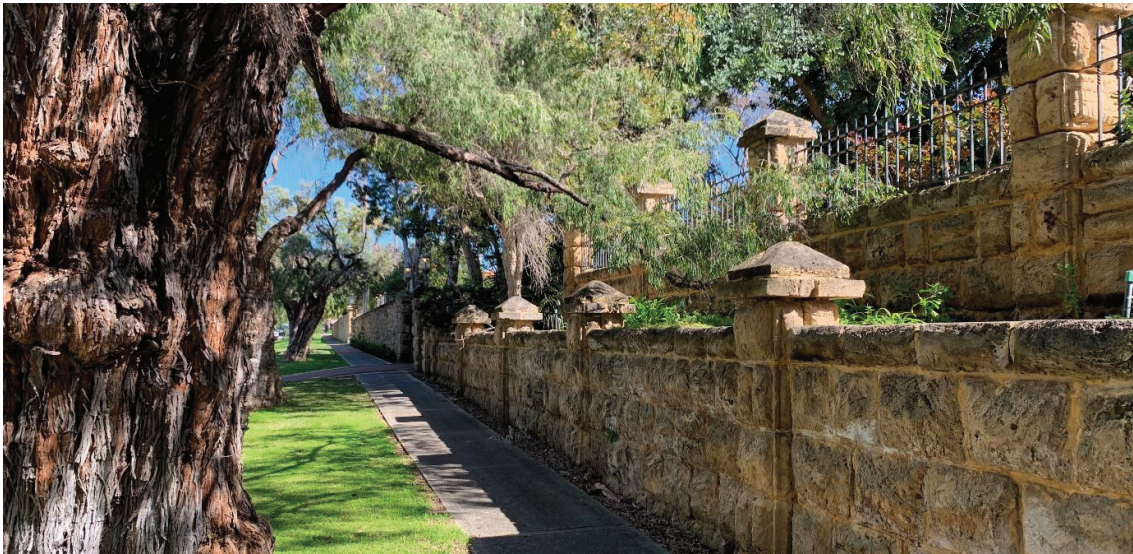
Photograph 2: Solid 'Pillow Face' limestone front walls at No.150 Forrest Street, with terraced landscaping and open fencing.
