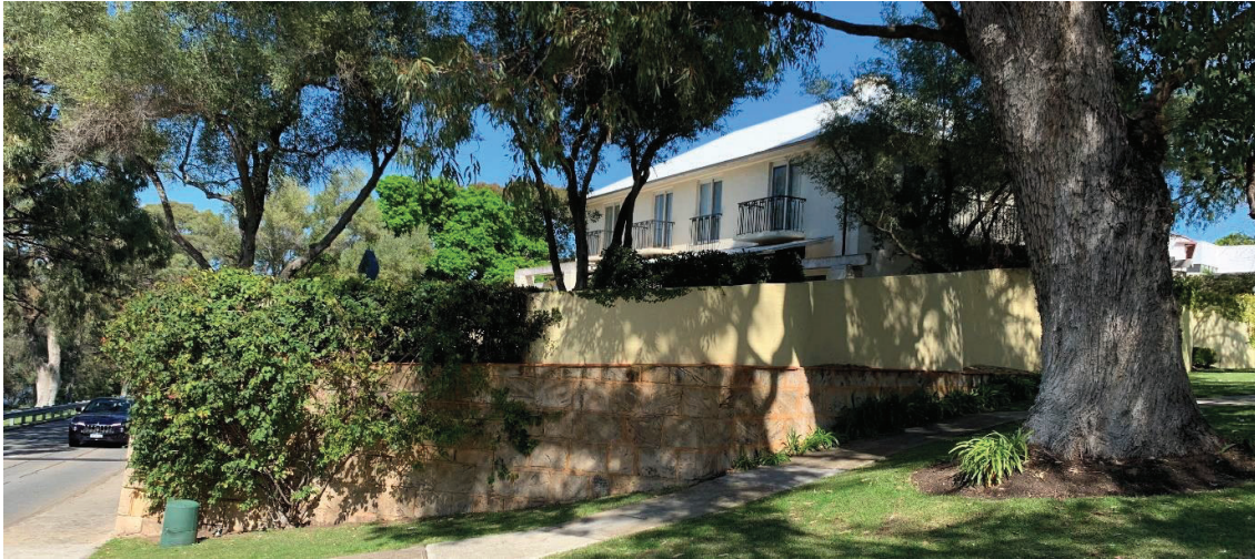
Photograph 3: No.16 The Esplanade, with a solid truncated wall fronting The Esplanade and Forrest Street.
