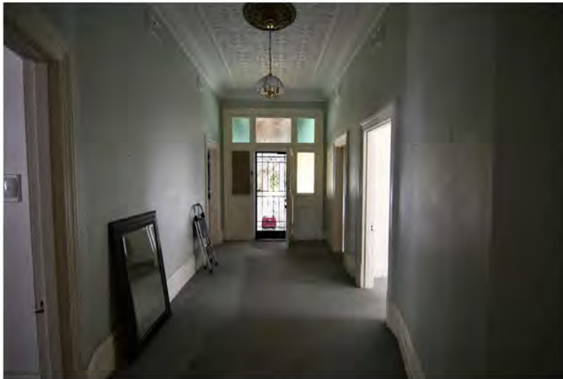
Photograph 12: Entrance Hall looking toward the front door. Griffiths Architects, September 2021.
