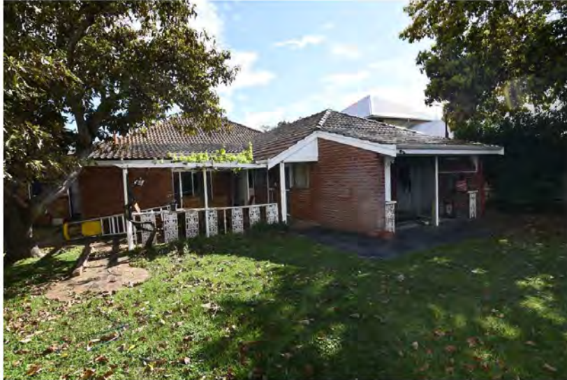
Photograph 11: Rear of the house looking north. Griffiths Architects, September 2021.
