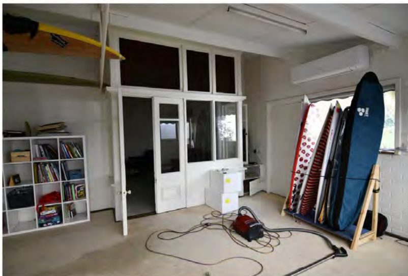
Photograph 19: An internal view showing the detail of the dining room bay. Griffiths Architects, September 2021.
