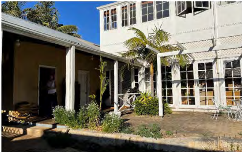
Photograph 08: Looking northeast showing the western courtyard, western extension and rear of the double storey portion of the residence. The enclosing shroud will be removed and replaced in a sympathetic new shroud. Griffiths Architects November 2021.
