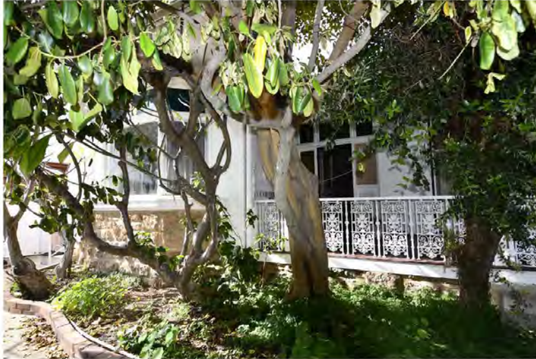
Photograph 7: Front entrance and bay window to bedroom 1. The balustrade is not original and clashes with the turned posts. Griffiths Architects, September 2021.
