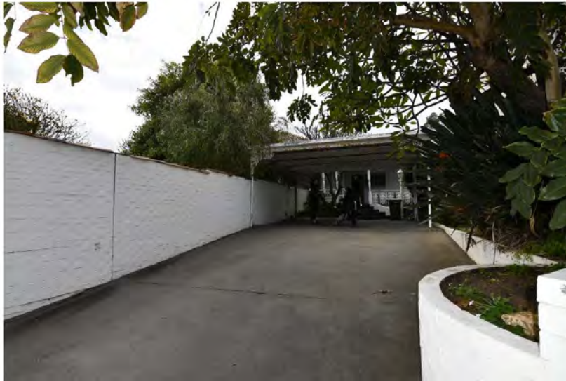
Photograph 4: 22 Irvine Street from the driveway. Griffiths Architects, September 2021.
