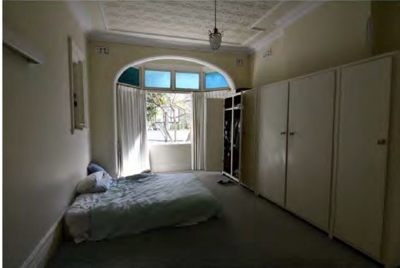
Photograph 14: Bedroom 1 looking north, with robes sourcing the fireplace. Griffiths Architects, September 2021.
