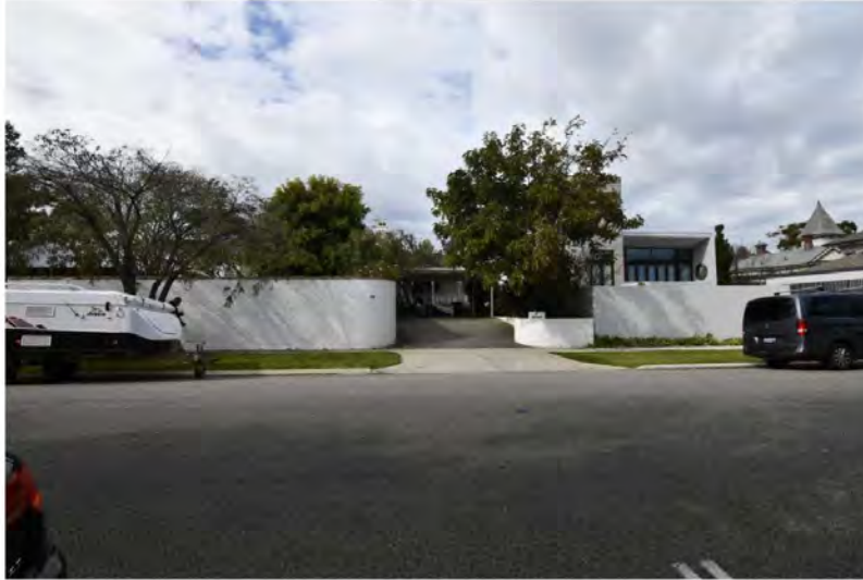
Photograph 3: 22 Irvine Street as it presents from the street. Griffiths Architects 2021.
