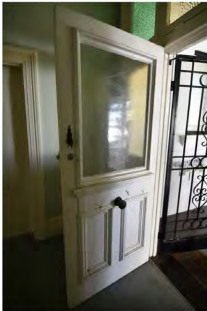
Photograph 22: The front door of 22 Irvine Street. Griffiths Architects, September 2021.
