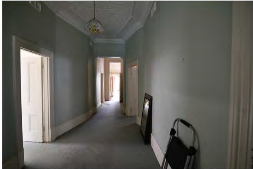
Photograph 13: Internal view of the hallway looking south. Griffiths Architects, September 2021.
