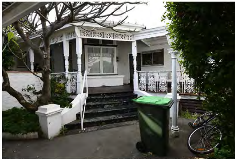
Photograph 6: The entrance steps, front verandah and bay window to formal lounge, and on the right is the later sleepout. Griffiths Architects, September 2021.
