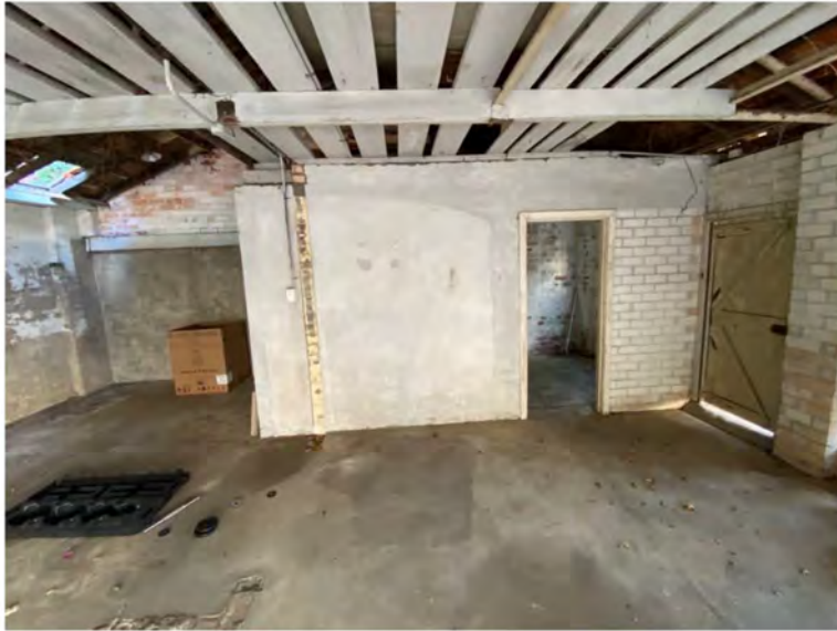
GARAGE INTERNAL | VIEW LOOKING NORTH
