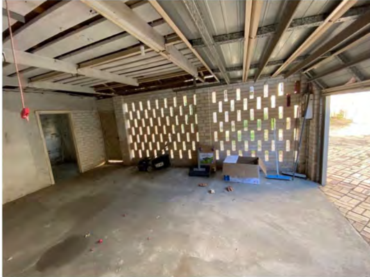
GARAGE INTERNAL | VIEW LOOKING EAST
