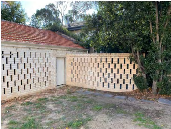
GARAGE | VIEW LOOKING NORTH INCLUDING BRICK WALL TO BE REMOVED
