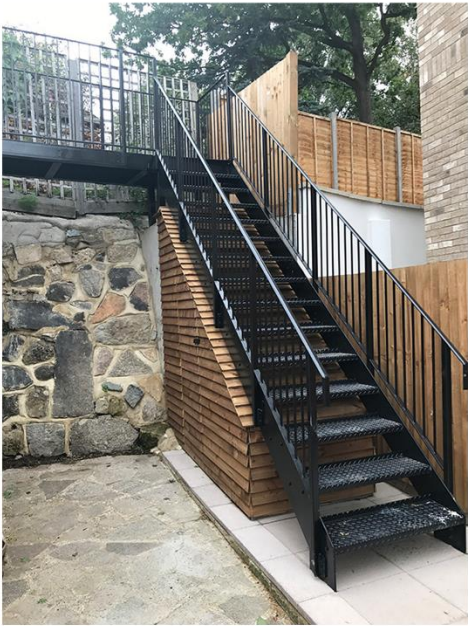
Steel Stair and Balustrade
