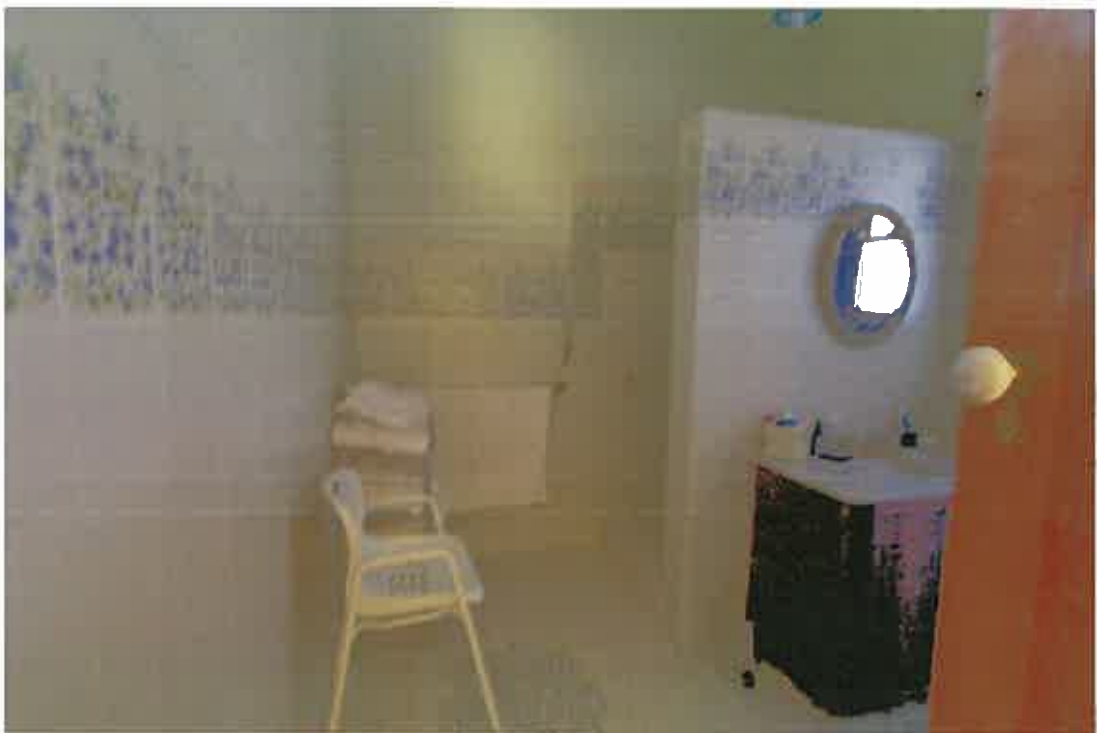
Photograph 12: Bathroom Griffiths Architects (2015)
