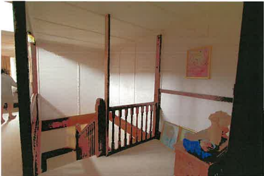
Photograph 14: Staircase from first floor landing Griffiths Architects (2015)
