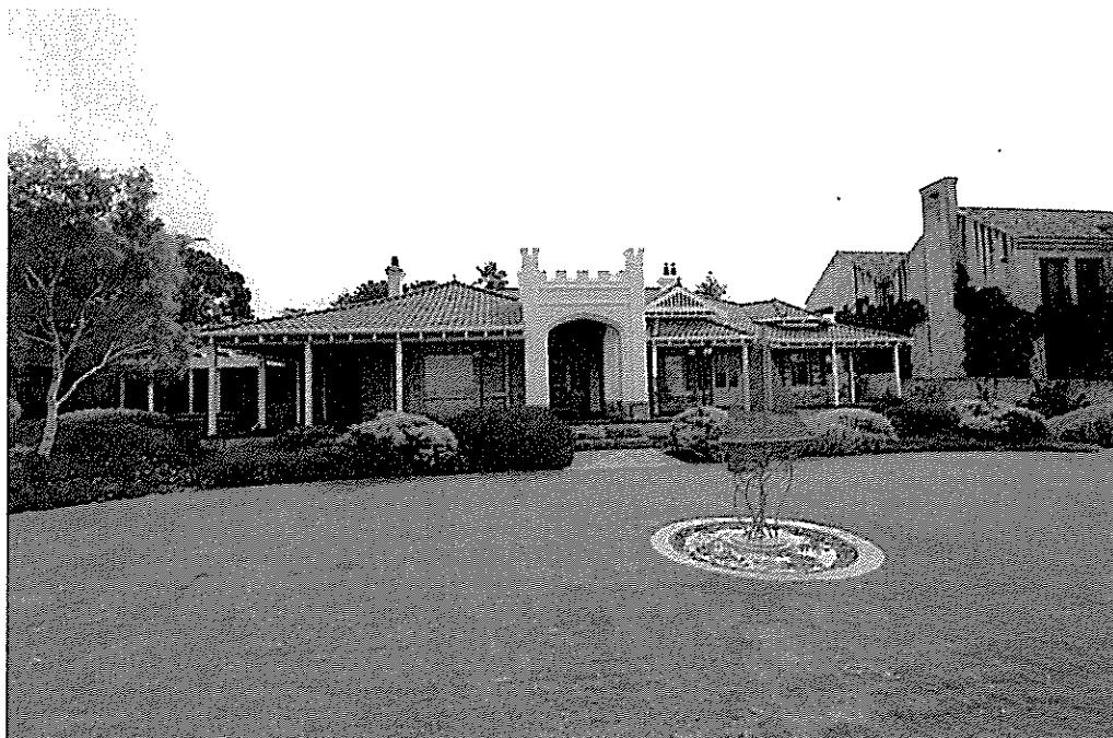
East elevation, indicating the 1927 entry, the added bay window to the left and change in gable treatments.
