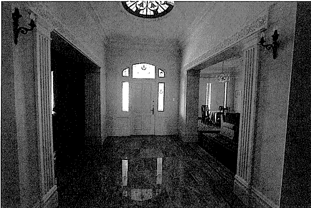
Hall looking east (Room 2) Floors, ceilings, cornices and openings are replacements.
