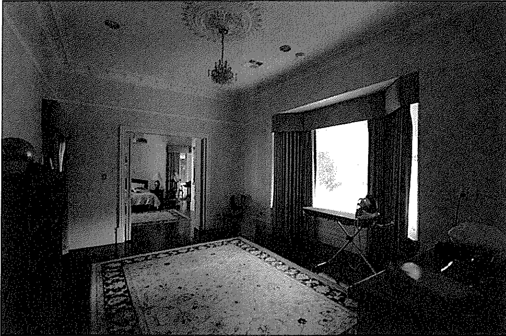
Retreat (Room 10). Although the main walls are part of the original house, it has been modified substantially, including the addition of the bay window to the right.
