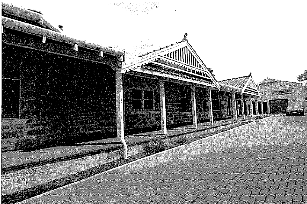
North side of the house. The verandah is a replacement and the gables to the verandahs a later addition.
