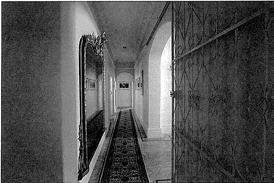
Corridor looking north. Floors, ceilings and cornices are replacement material.
