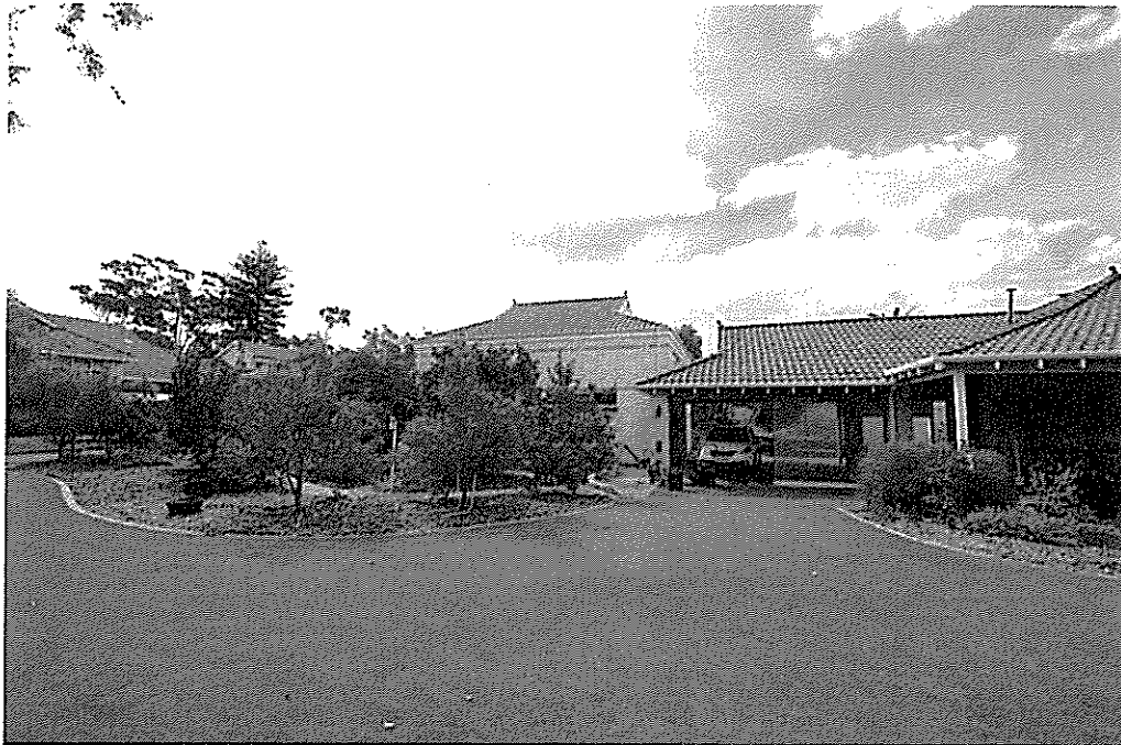
All the work in this photograph is a late addition.
