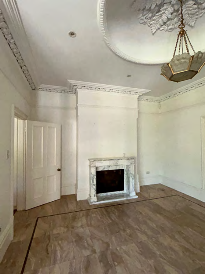
Image 97. View north-east in 1986 Dining Room, capturing contemporary marble chimneypiece, stone tile floor and pierced-work ceiling mouldings. (Source: PA 2023)
