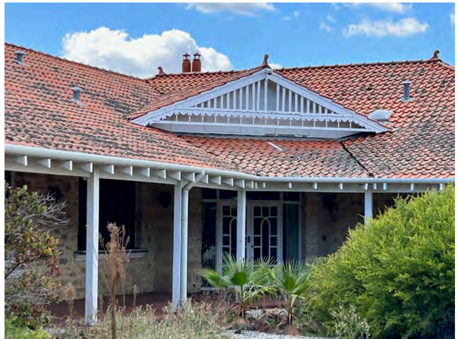
Image 44. View north-west towards 1986 'Dining Room'. Captures roof and verandah from 1986 construction. (Source: PA 2023)
