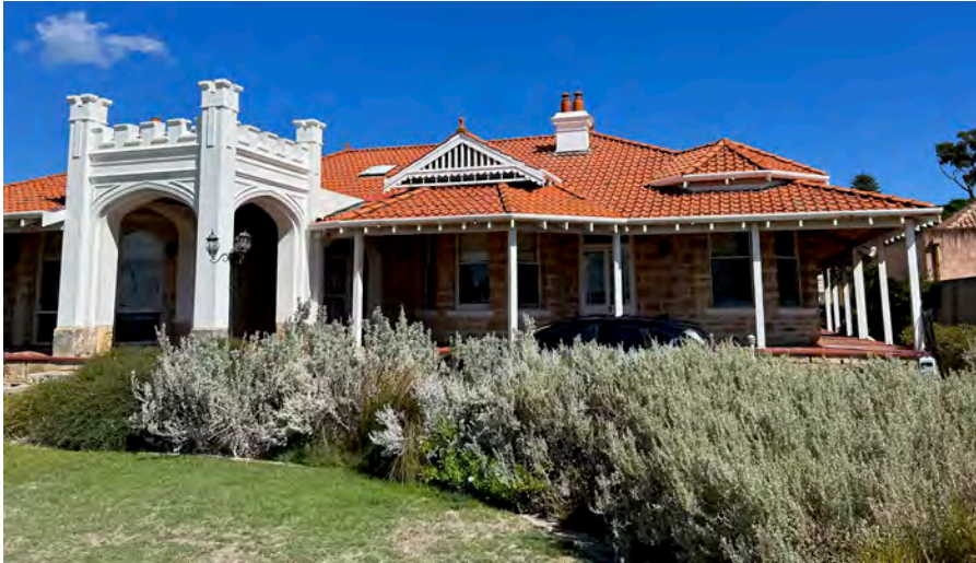
Image 03. View west towards eastern facade of 52 The Esplanade, capturing 1927 Post-War Gothic portico and 1897 Federation Queen Anne bay windows. Note 1986 roof and verandah. (Source: PA 2023)
