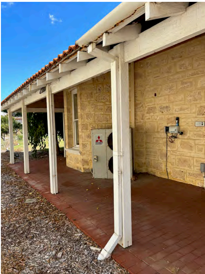
Image 33. View west along south facade of 1986 southern extension. (Source: PA 2023)
