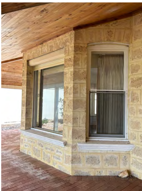
Image 30. View south towards bay window of 1986 addition, located south of 1927 'Dining Room'. (Source: PA 2023)
