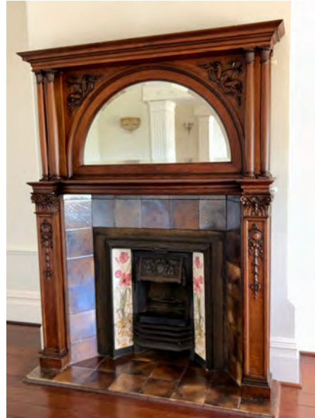
Image 57. Cast iron fireplace with timber mantle to northern front room. (Source: PA 2023)
