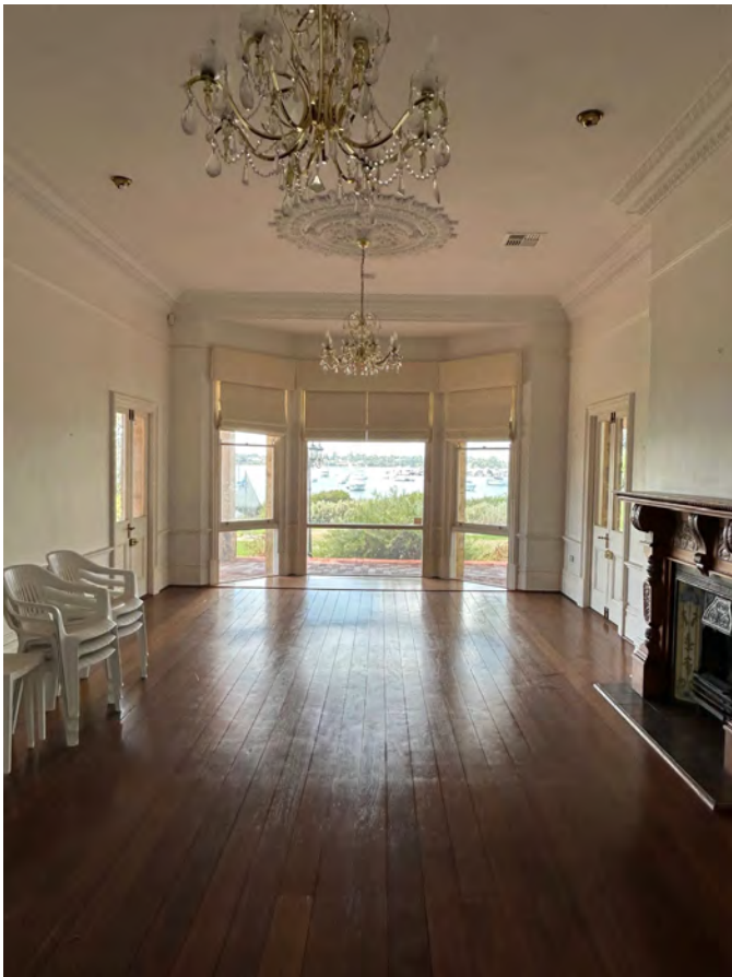
Image 62. View east towards bay window of 1927 Dining Room, capturing cast iron fireplace with timber chimneypiece. Note c.1986 plasterwork to ceiling. (Source: PA 2023)
