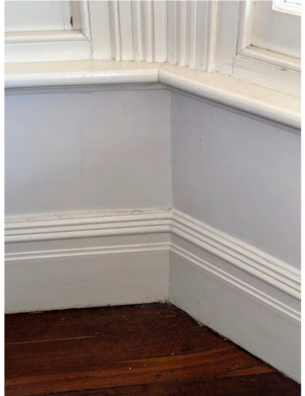
Image 73. Detail of timber skirting and timber window frames and sill. (Source: PA 2023)
