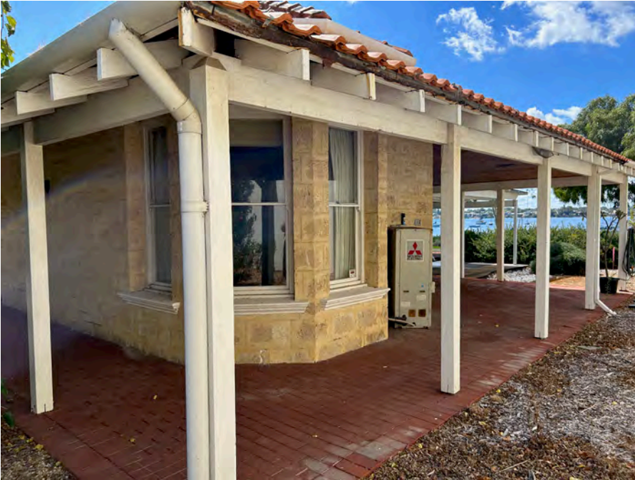
Image 32. View north-east towards The Esplanade from south-east boundary. (Source: PA 2023)
