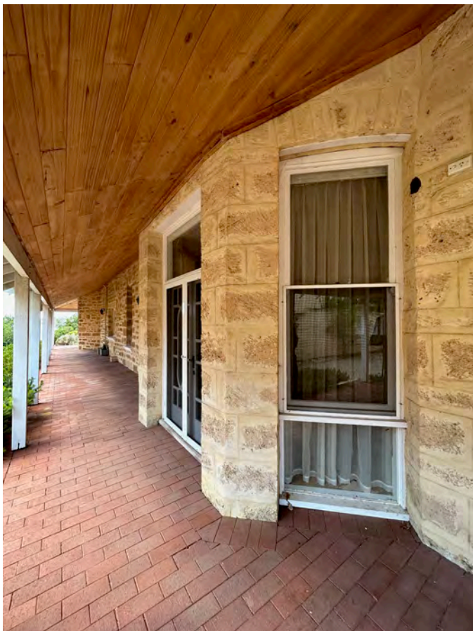
Image 17. View south-west towards bay window and double entry doors of 1986 addition. Note difference between stone quality of 1897 and 1986 fabric. (Source: PA 2023)
