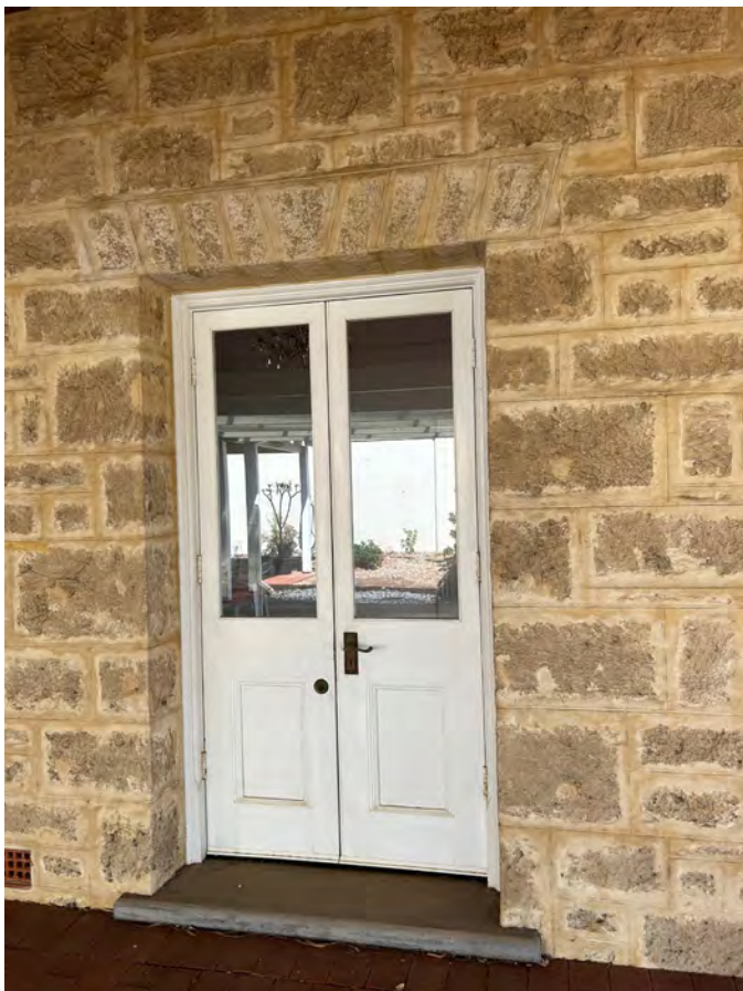
Image 26. Detail image of southern double door to 1927 'Dining Room'. (Source: PA 2023)
