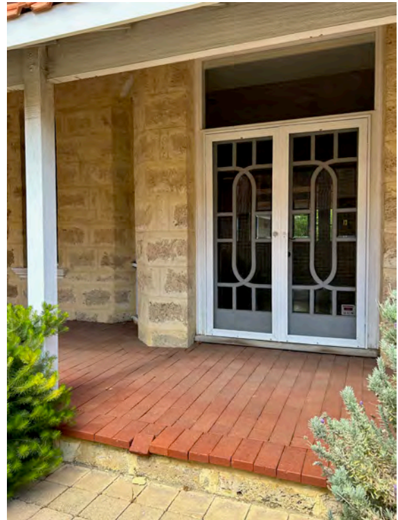
Image 18. Detail image of northern double entry doors en-sconced in a bay window of the 1986 build. (Source: PA 2023)
