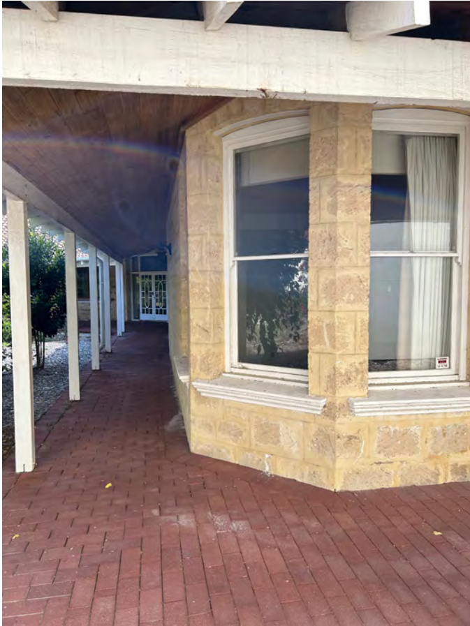
Image 35. View north along west verandah of 1986 southern extension. (Source: PA 2023)
