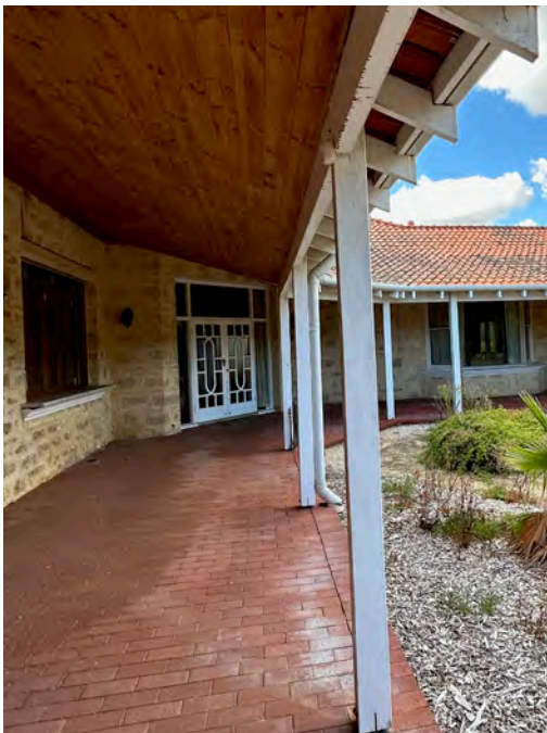
Image 43. View east along southern verandah of northern wing. (Source: PA 2023)
