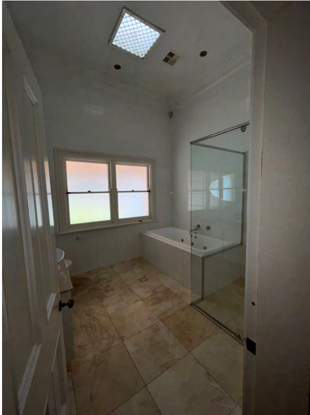
Image 76. View north into Bathroom. Note windows in location of original main entrance to 1897 cottage. (Source: PA 2023)
