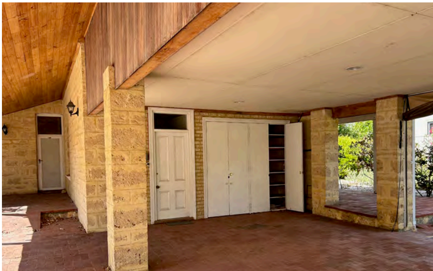
Image 49. View east towards western (back) entry to 1986 addition via undercover car parking area. (Source: PA 2023)
