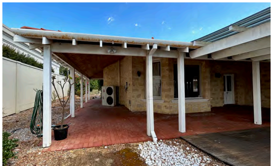
Image 31. View west towards 1986 addition, located south of 1927 'Dining Room'. (Source: PA 2023)
