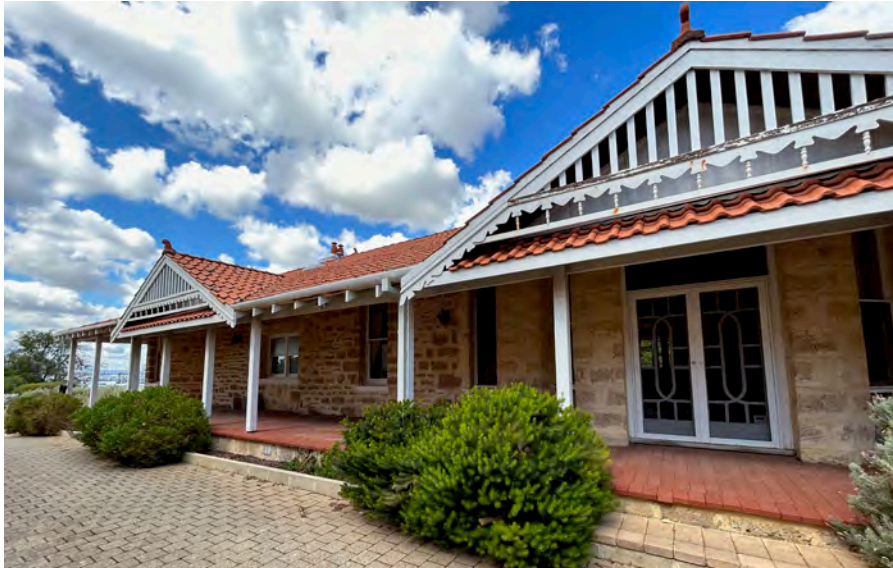
Image 10. View south-east of north facade, capturing 1986 addition to 1897 fabric. Note 1986 roof and verandah. (Source: PA 2023)
