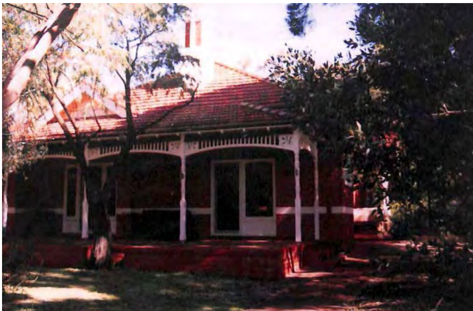
Fig 16. 58 The Esplanade , before demolition. (Source: Shire of Peppermint Grove)
