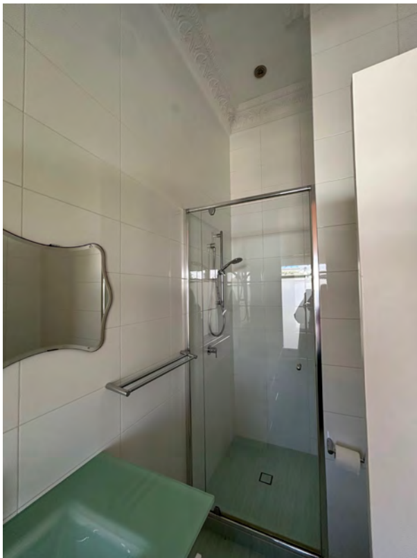
Image 92. View into Ensuite of western 1986 Bedroom addition. (Source: PA 2023)
