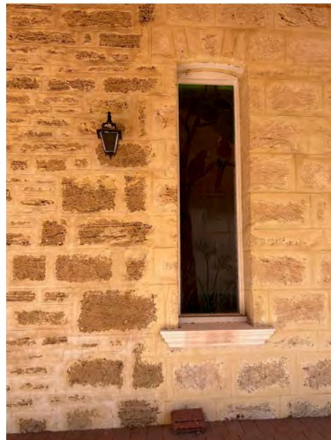
Image 16. Detail image of stained glass window that aligns with the internal stairs down to the cellar. Note the difference in the Cottesloe limestone of the 1897 fabric and Carabooda limestone of the 1986 addition. (Source: PA 2023)
