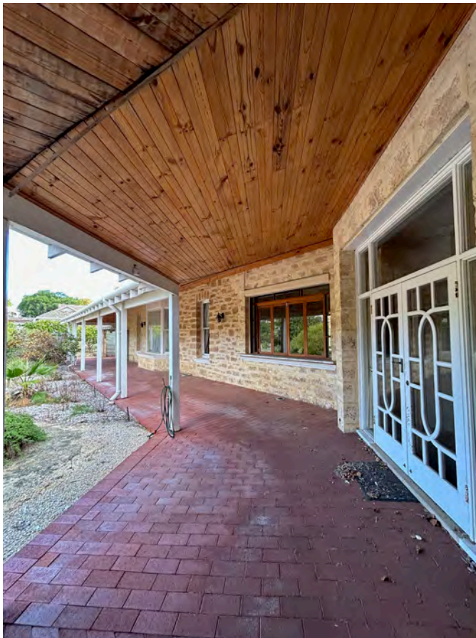
Image 37. View north-west along western verandah. (Source: PA 2023)
