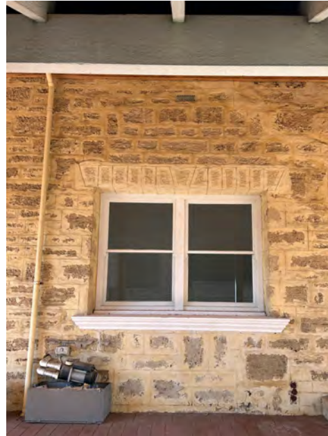
Image 13. Detail image of window installed at location of original main entry door to 1897 cottage. Note difference between Cottesloe limestone and more recently layed Carabooda limestone infill. (Source: PA 2023)
