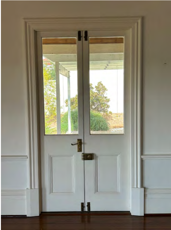
Image 64. Timber double doors to 1927 Dining Room. (Source: PA 2023)
