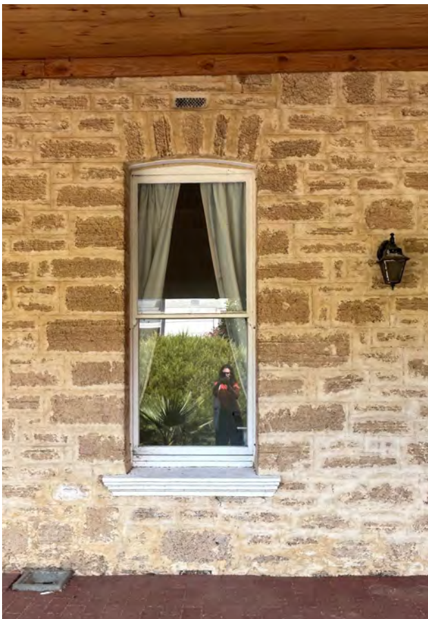
Image 40. Detail image of contemporary window and bar into Kitchen. Captures difference in Cottesloe limestone to lower wall and Carabooda limestone around window. (Source: PA 2023)
