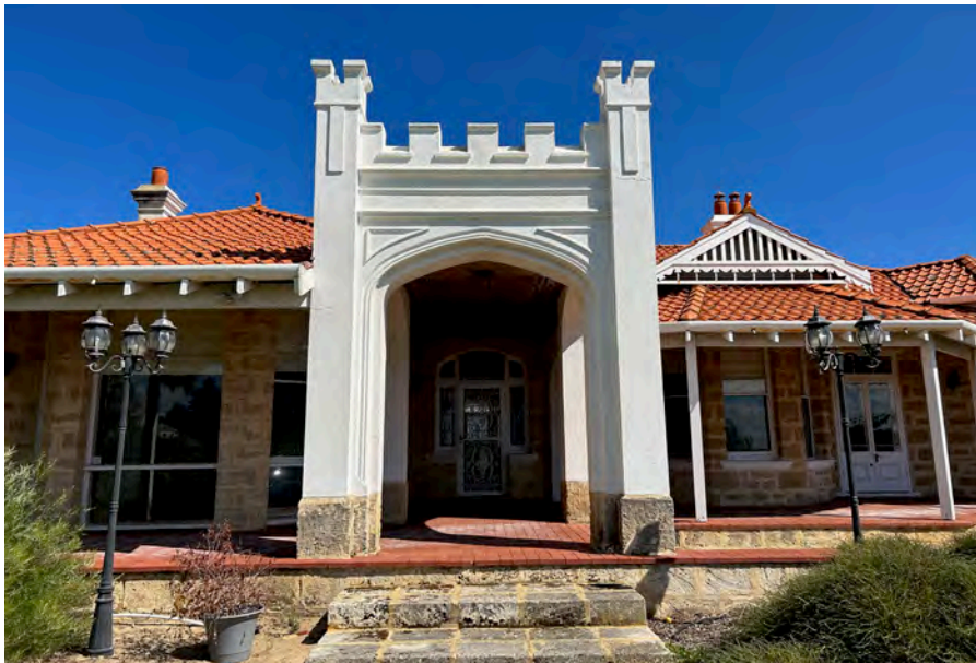
Image 04. View west towards main entry, through the 1927 Post-War Gothic portico. Note 1897 fabric to the right of the image. (Source: PA 2023)
