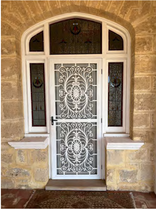
Image 06. Main entry doorway (From 1927 addition. Noted as original 'Existing Doorway and Sidelights' in 1945 floor plan.) 1986 doors, sidelights and frame. (Source: PA 2023)
