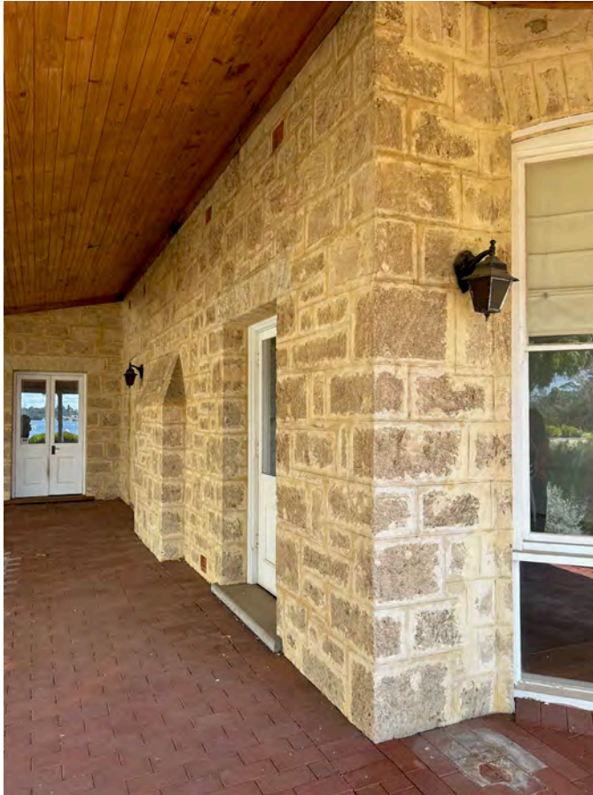
Image 25. View west along southern wall of 1927 'Dining Room' towards. (Source: PA 2023)
