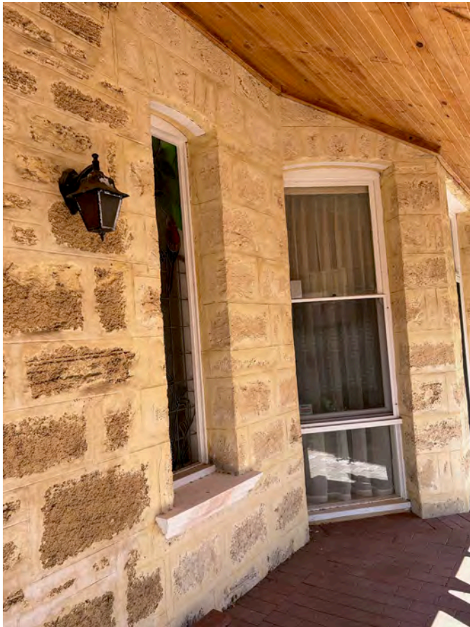
Image 17. View south-west towards bay window and double entry doors of 1986 addition. Note difference between stone quality of 1897 and 1986 fabric. (Source: PA 2023)
