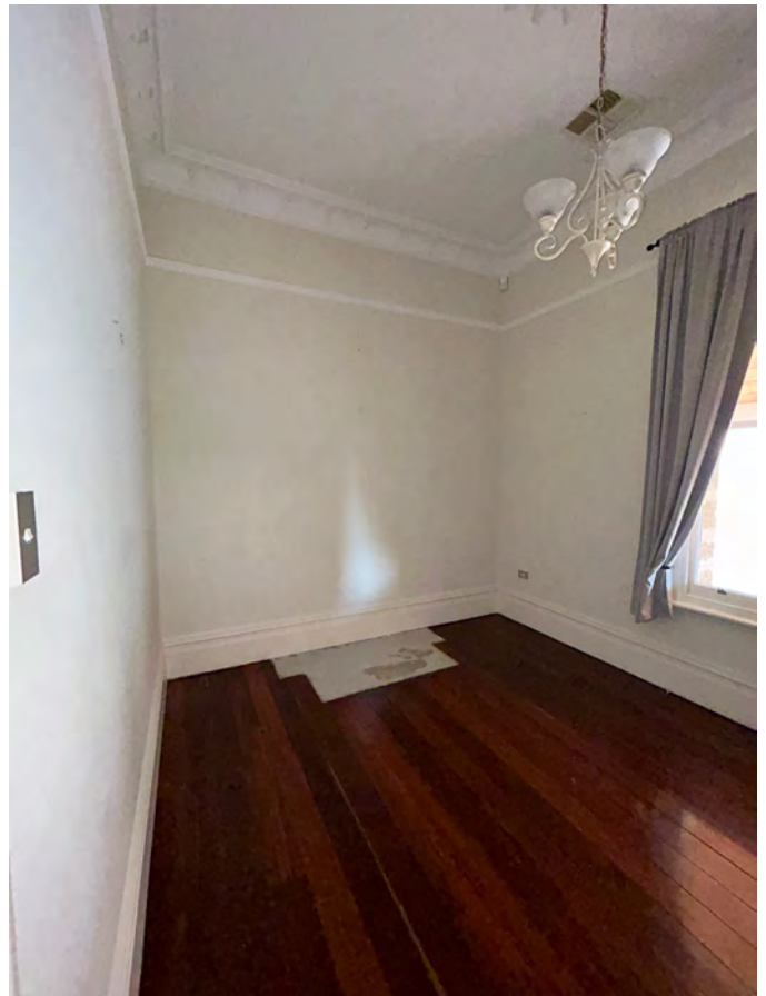
Image 78. View north-west from doorway into Bedroom. Note remnant hearthstone of removed fireplace. (Source: PA 2023)
