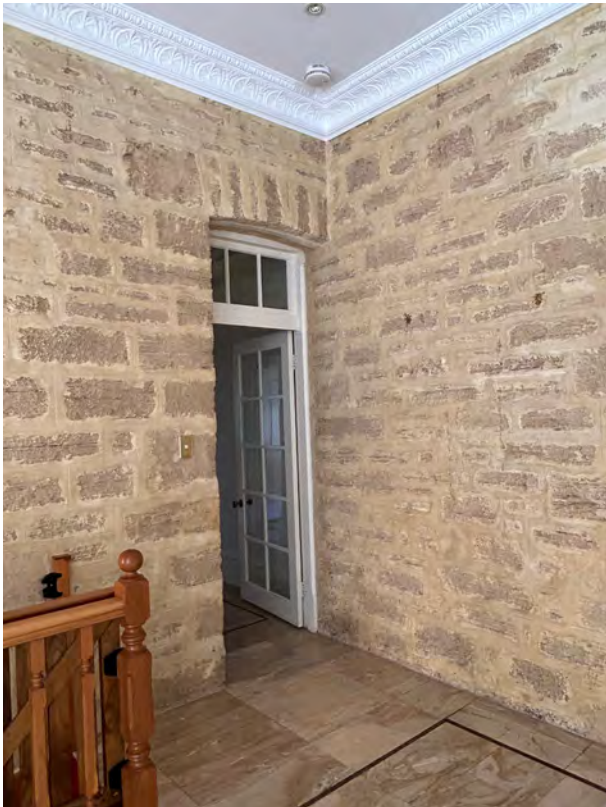
Image 83. View east north towards door at western termination of corridor from Lounge Room. Note exposed limestone walls with stone lintel (c.1895) over doorway and ornamental cornice, stone floor tiles and timber balustrade (c.1986) to stairs leading down to Cellar. (Source: PA 2023)
