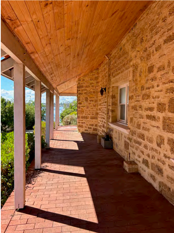
Image 13. Detail image of window installed at location of original main entry door to 1897 cottage. Note difference between Cottesloe limestone and more recently layed Carabooda limestone infill. (Source: PA 2023)
