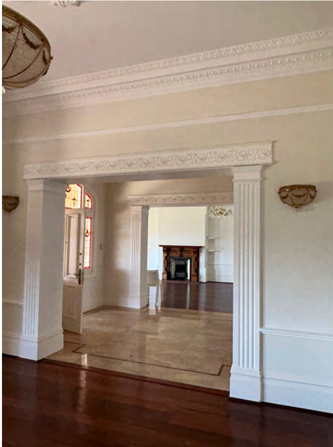
Image 61. Detail image of 1986 decorative pilaster and moulding to flat arch. (Source: PA 2023)
