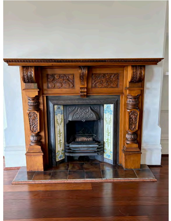
Image 65. Cast iron fireplace with timber chimney-piece to southern wall of 1927 Dining Room. (Source: PA 2023)
