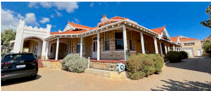
Image 02. View west towards eastern facade of 52 The Esplanade, capturing 1927 Post-War Gothic portico, 1897 Federation Queen Anne bay windows, 1986 extension and 1996 Garage behind. Note 1986 roof and verandah. (Source: PA 2023)
