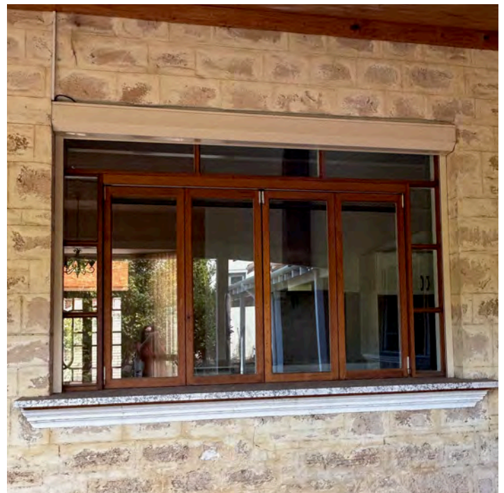
Image 40. Detail image of contemporary window and bar into Kitchen. Captures difference in Cottesloe limestone to lower wall and Carabooda limestone around window. (Source: PA 2023)
