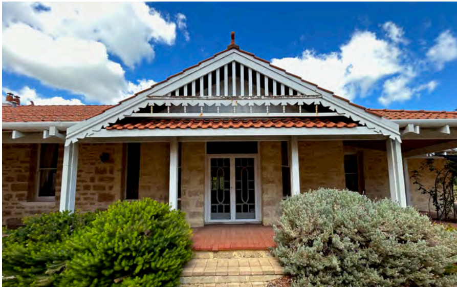
Image 11. View south towards northern facade, capturing double doors and bay windows under a gabled verandah roof of the 1986 addition. (Source: PA 2023)
