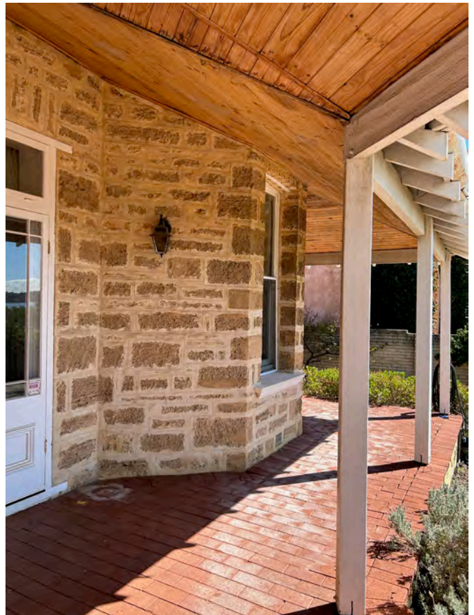
Image 09. Northern corner bay window from 1897 build. (Source: PA 2023)
