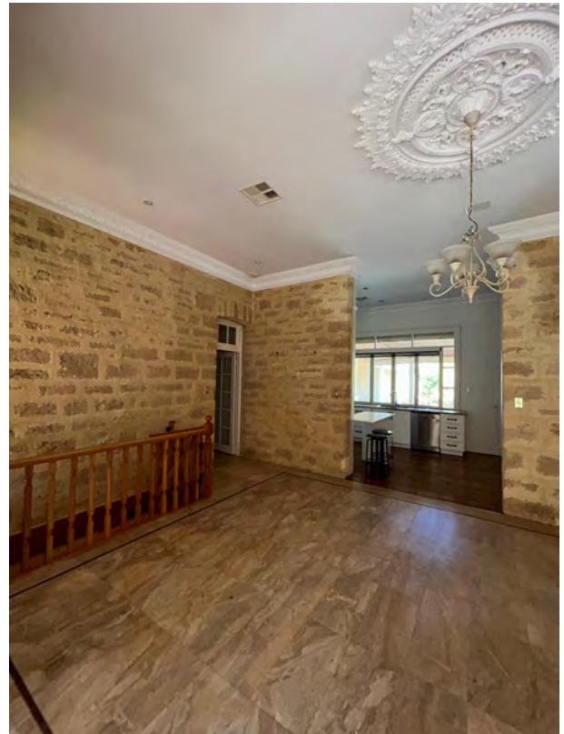
Image 84. View south-east towards Kitchen and door to western end of corridor. Note exposed limestone walls with stone lintel over doorway. Ornamental cornice, stone floor tiles and timber balustrade to stairs leading down to Cellar are from 1986 works. (Source: PA 2023)
