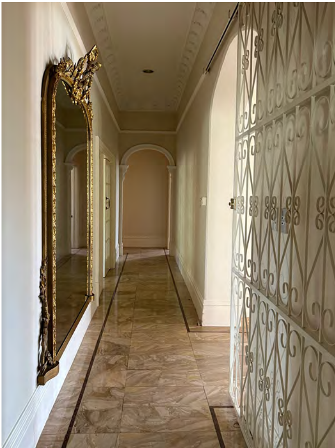
Image 68. View north along corridor from southern end, capturing the sliding security gate to behind the Gothic arch. (Source: PA 2023)
