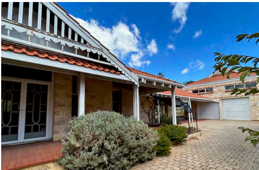
Image 12. View south-west towards 1986 addition and 1996 Garage. (Source: PA 2023)
