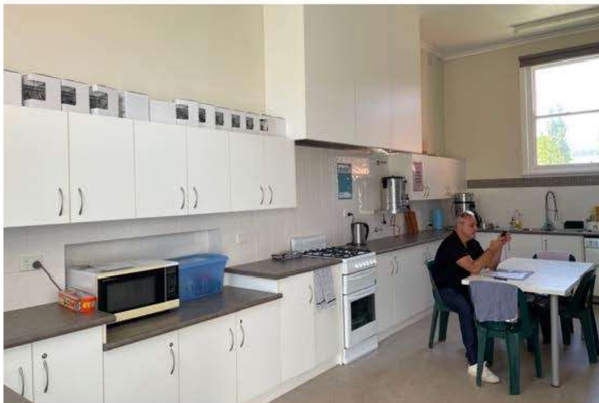
Photograph D6: The kitchen area which will become a store. Griffiths Architects February 2022
