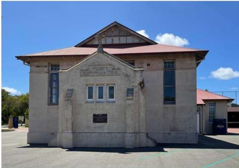
Photograph 01: West face of the church hall. Griffiths Architects February 2022
