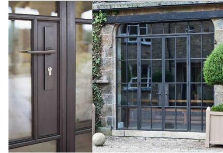
NEW REAR PAVILION FENESTRA - BRONZE FRAME, DOUBLE GLAZED WINDOWS & DOORS.
