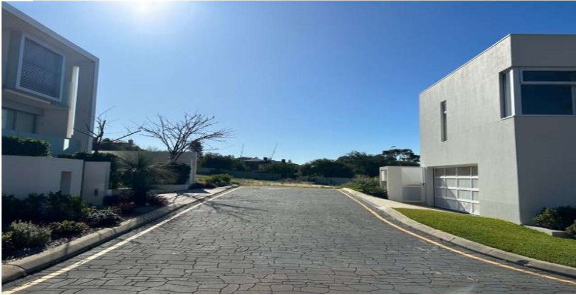
View to site from south at head of Bungalow Court
