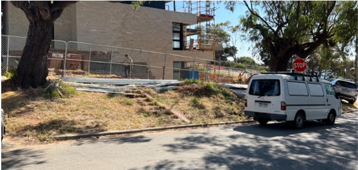
Figure 1: Condition of Existing Verge and Slope Characteristics
