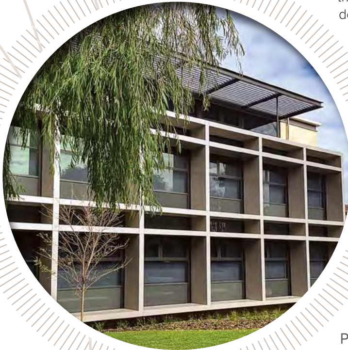
The PLC Music Room an example of commercial building work.
