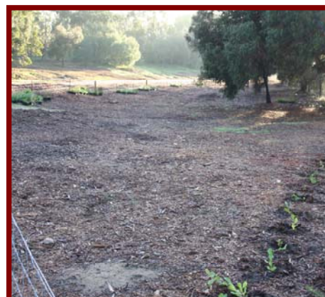
Wetland buffer being planted
